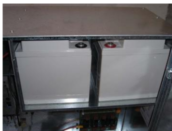
Figure 3 - 24 Vdc monoblocs series installation
